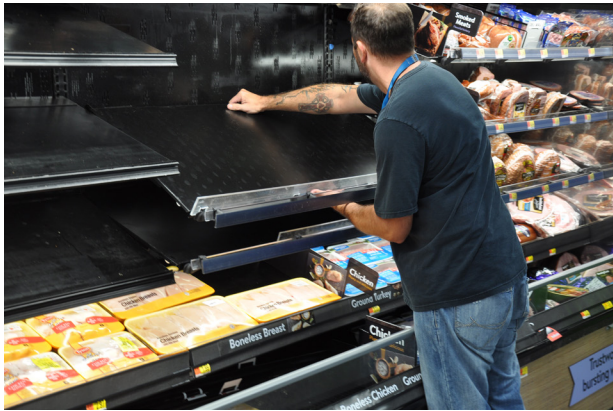
Installer retrofitting an Ecoblade shelf to an existing case.
